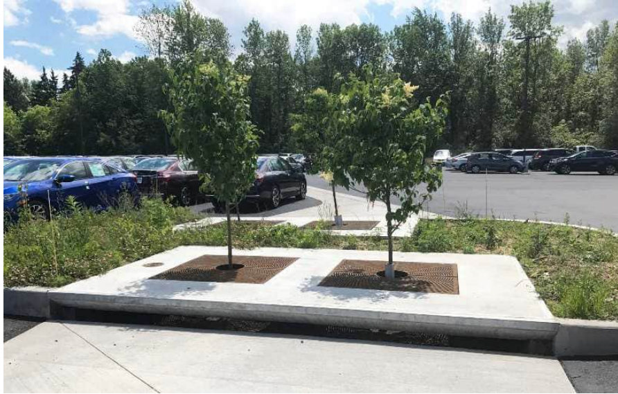
Figure 28 - Tree Filter Boxes (Source: Contech Engineered Solutions)
